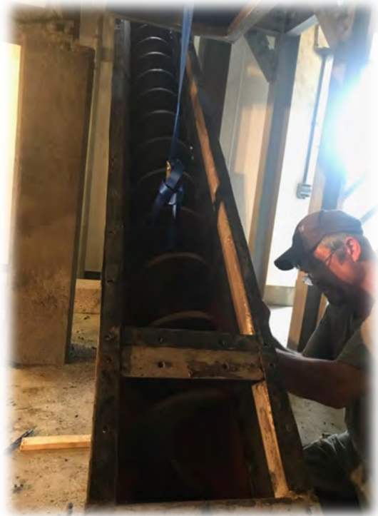
Photo 2 Randy working on liner installation
