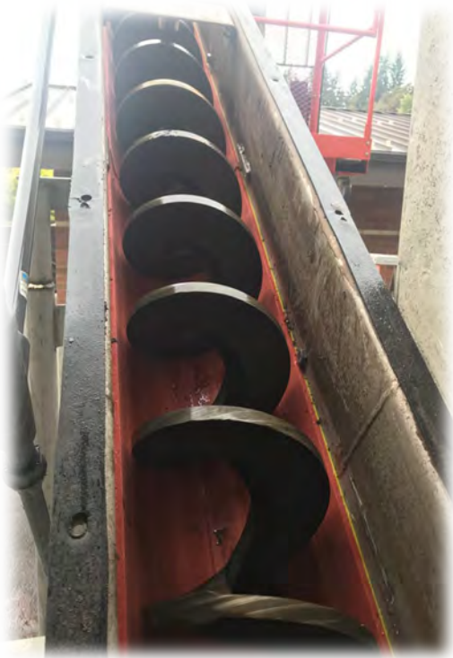
Photo 1 The new liner installed
