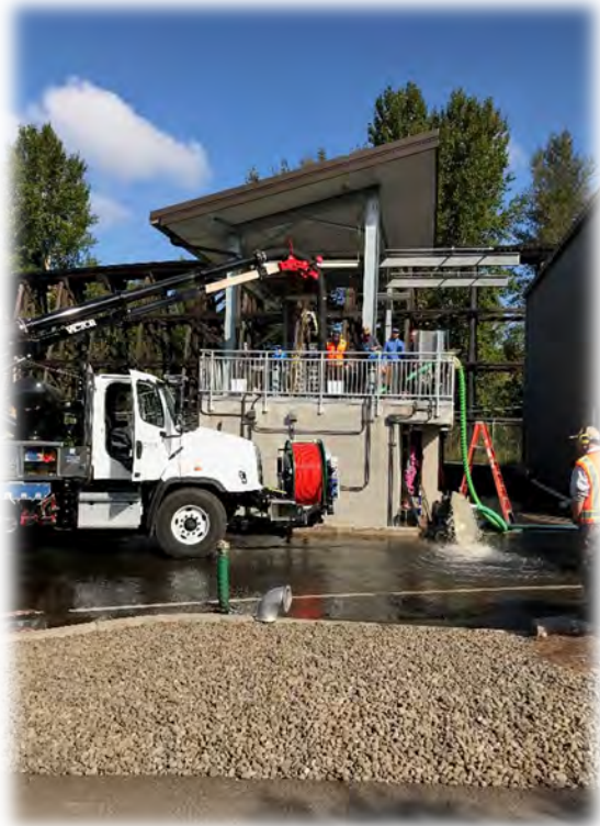
Photo 4 Pumping out the valve box
