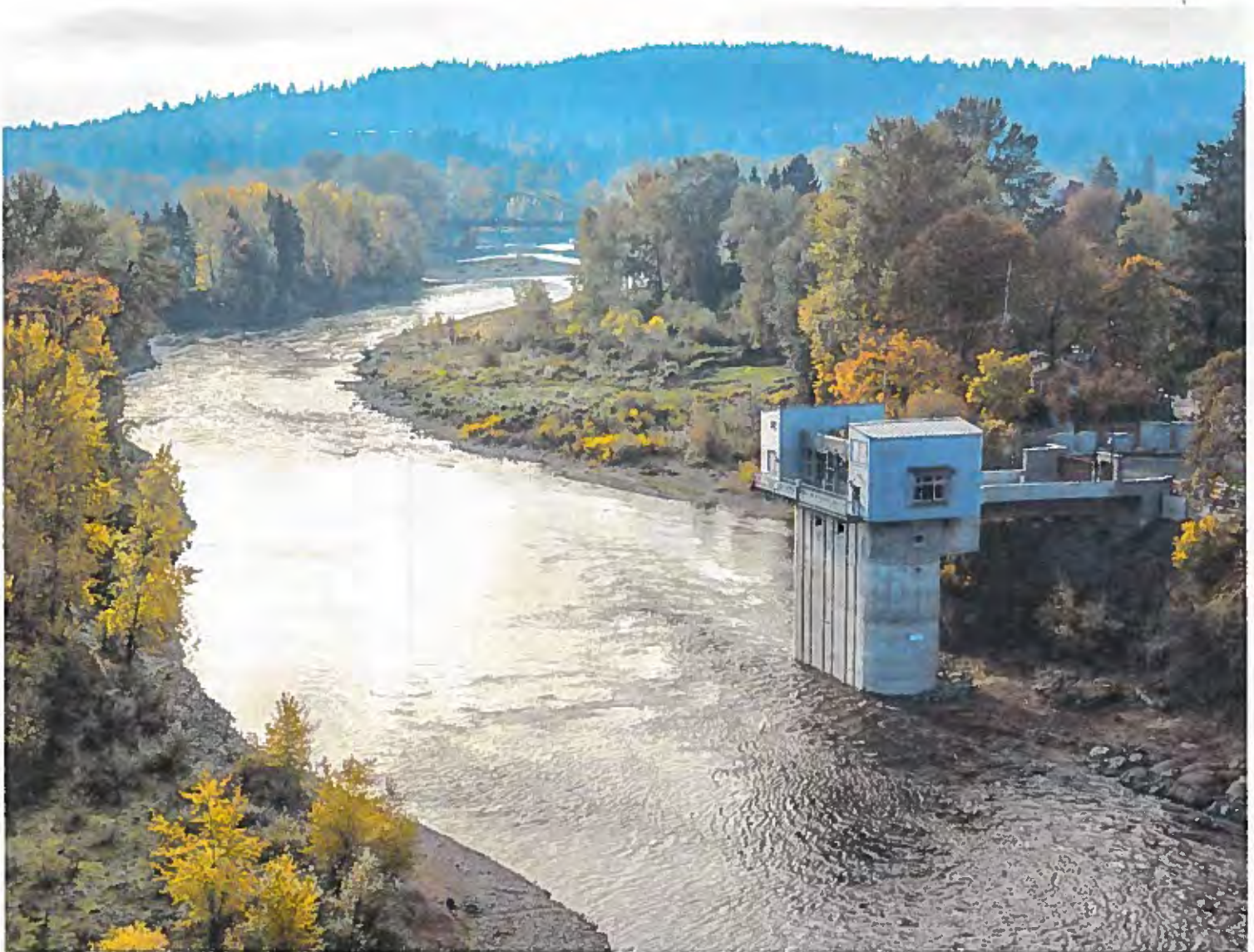
The Lake Oswego Tigard Water Partnership's river intake pump station on the Clackamas River
