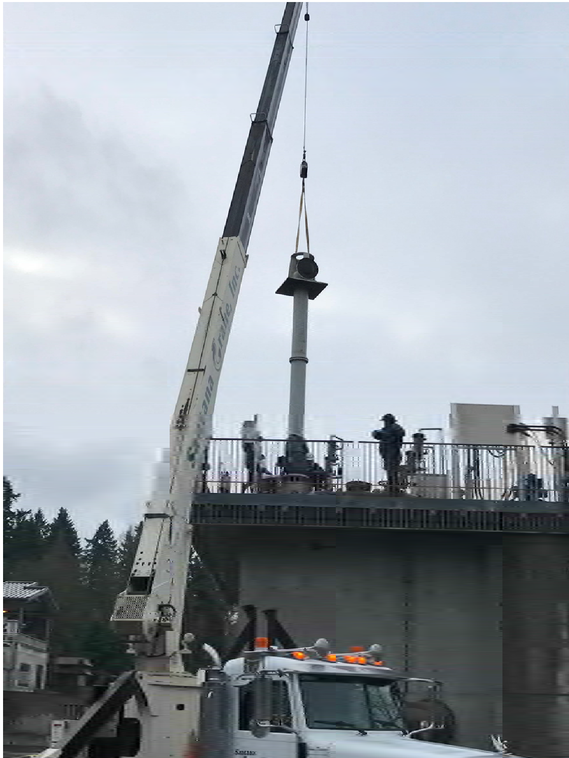
Photo 2 Installing Rebuilt Mixed Liquor Return pump.
