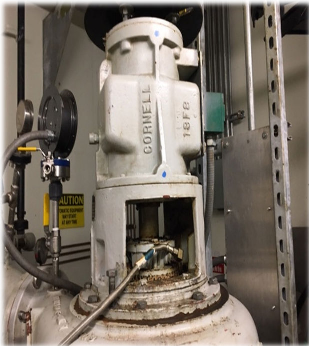
Pump Station #2 before painting.
