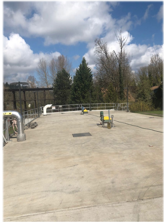
IBR after pressure wash
