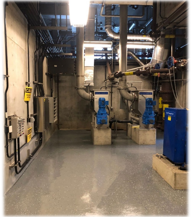
Headworks floor painting
