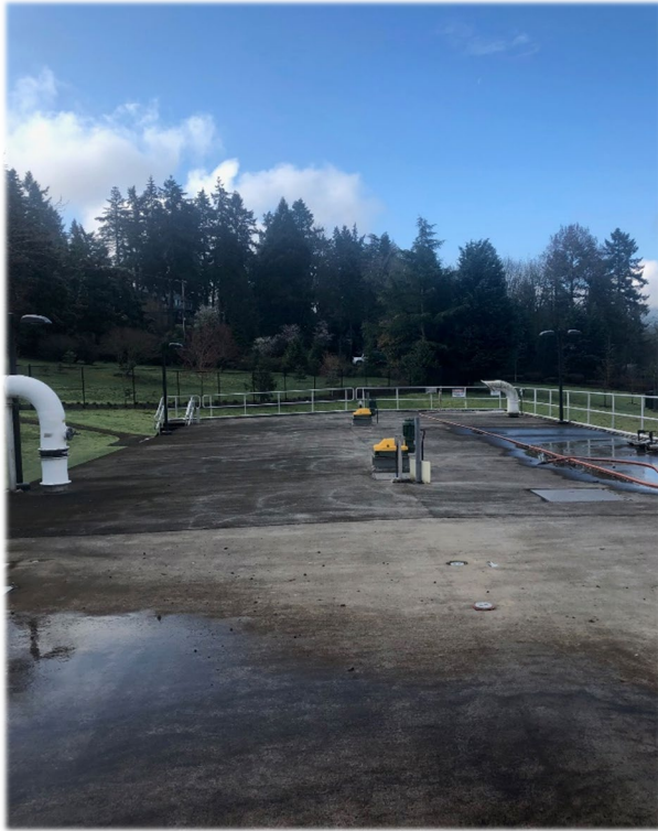
IBR before pressure wash
