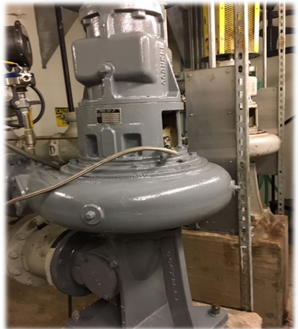
Pump Station #2 after painting
