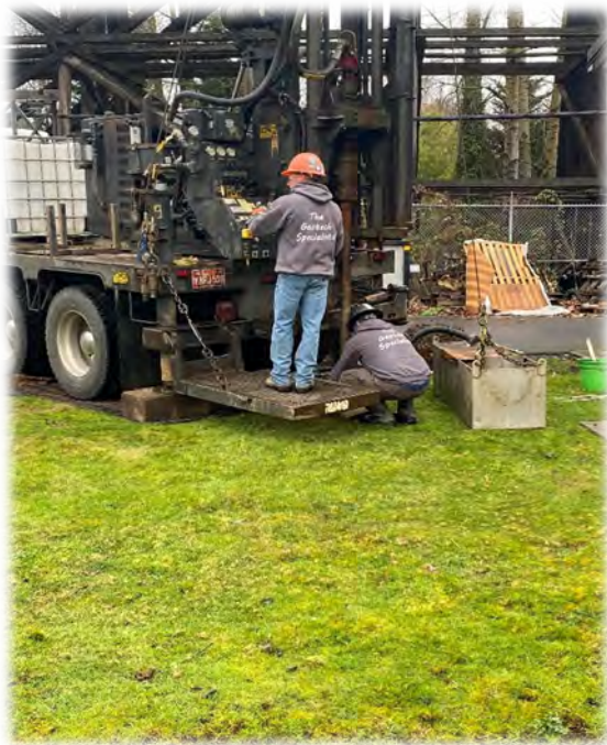
Potholing where the Filters are going.
