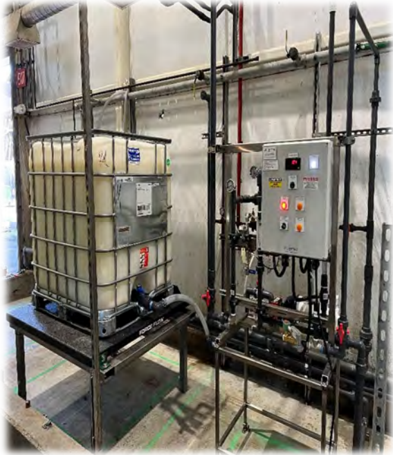
Permanent Polymer system install.
