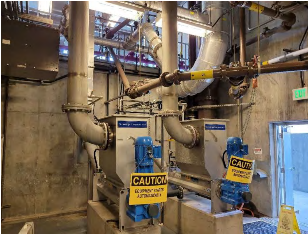
Figure 12. Screenings washer/compactors
