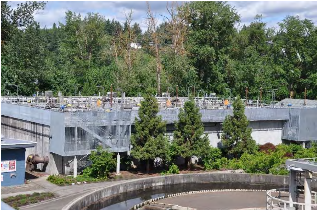
Figure 20. Aeration basin structure
