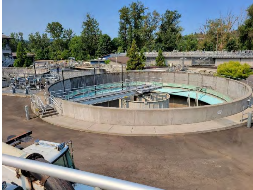
Figure 22. Original secondary clarifier
