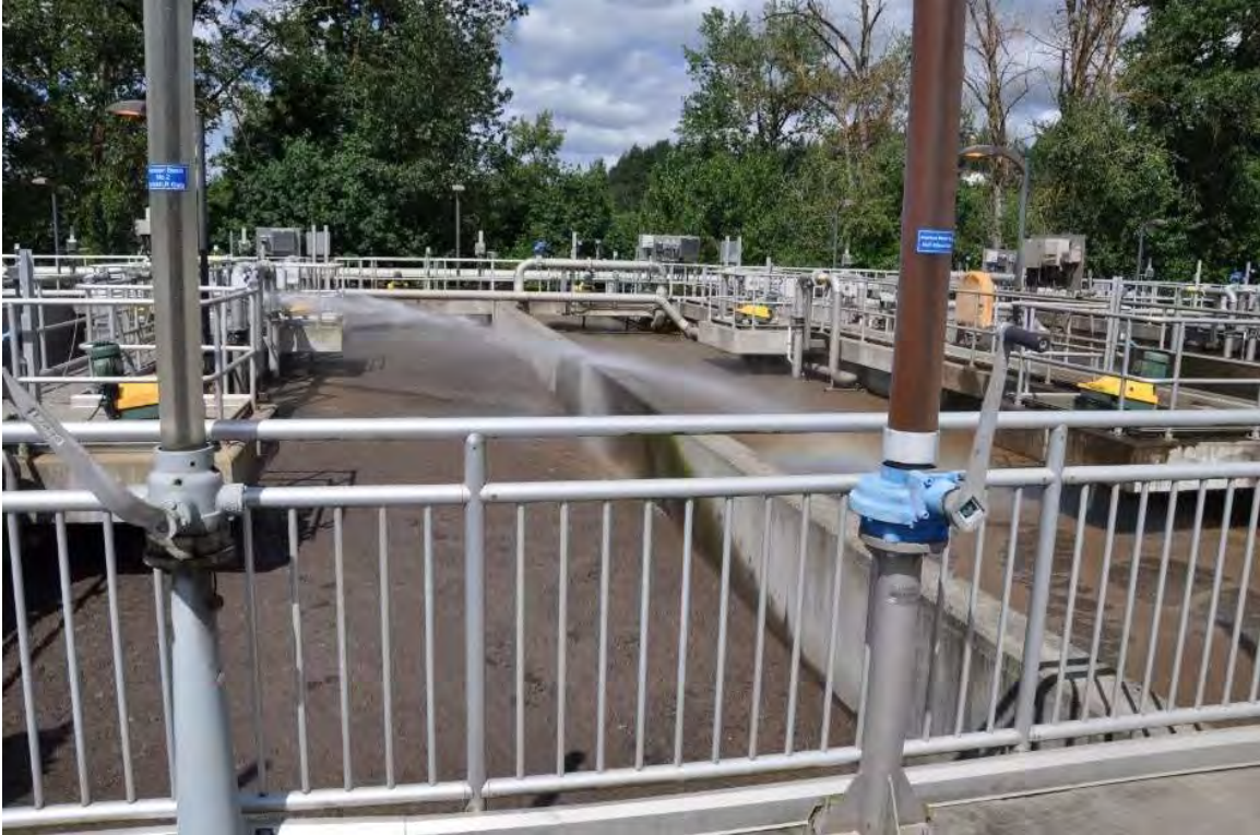
Figure 22. Aeration basin showing use of hoses for spray water
