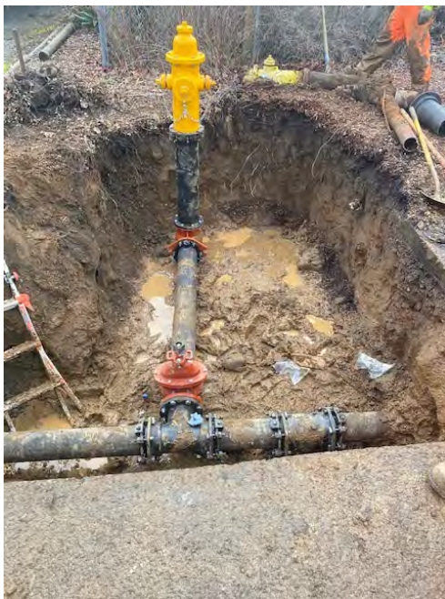
After New hydrant installation
