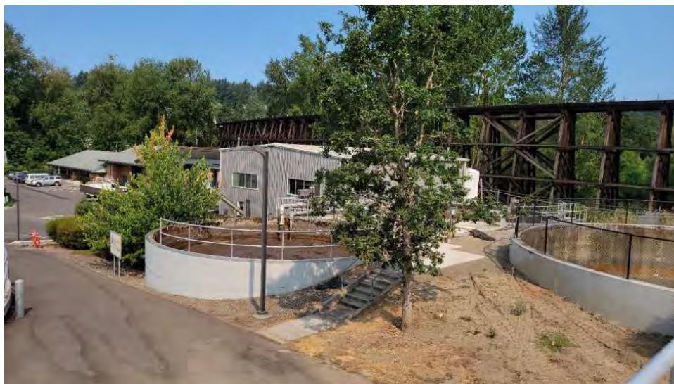
Figure 29. Circular aerobic digester
