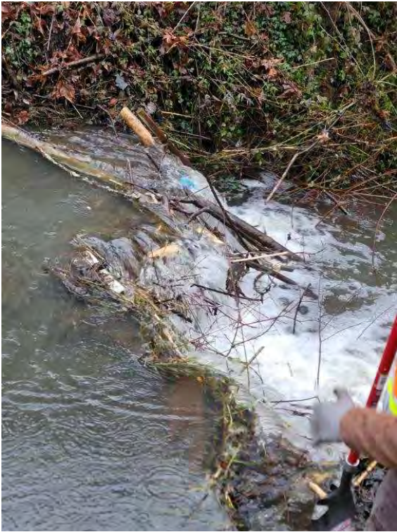
Beaver dam removal
