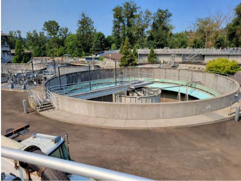
Figure 29. Original secondary clarifier
