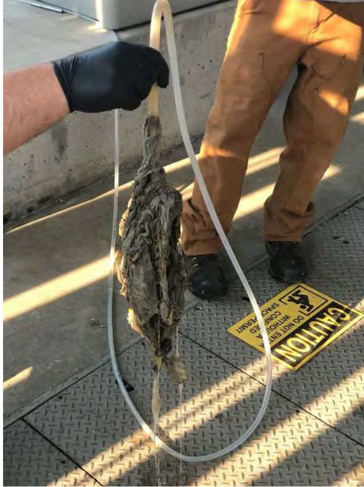
Figure 10. Debris accumulation on influent sampler suction strainer
