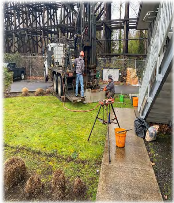
Geotechnical Potholing part 2.
