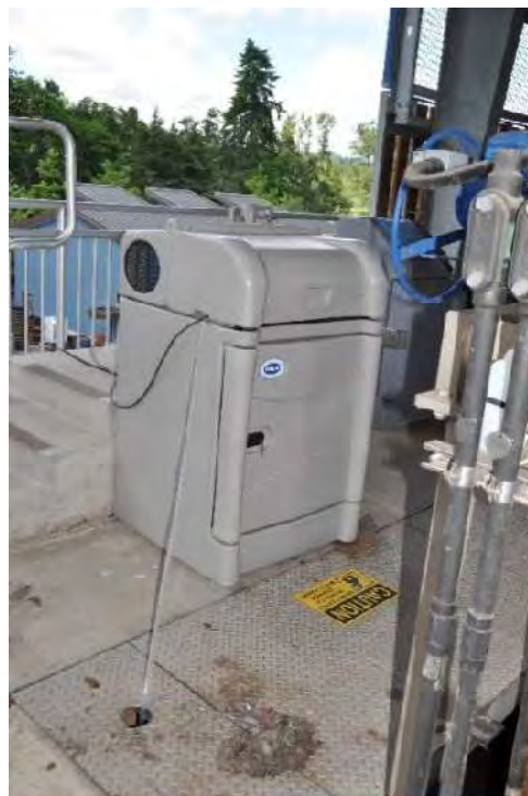
Figure 8. Influent composite sampler
