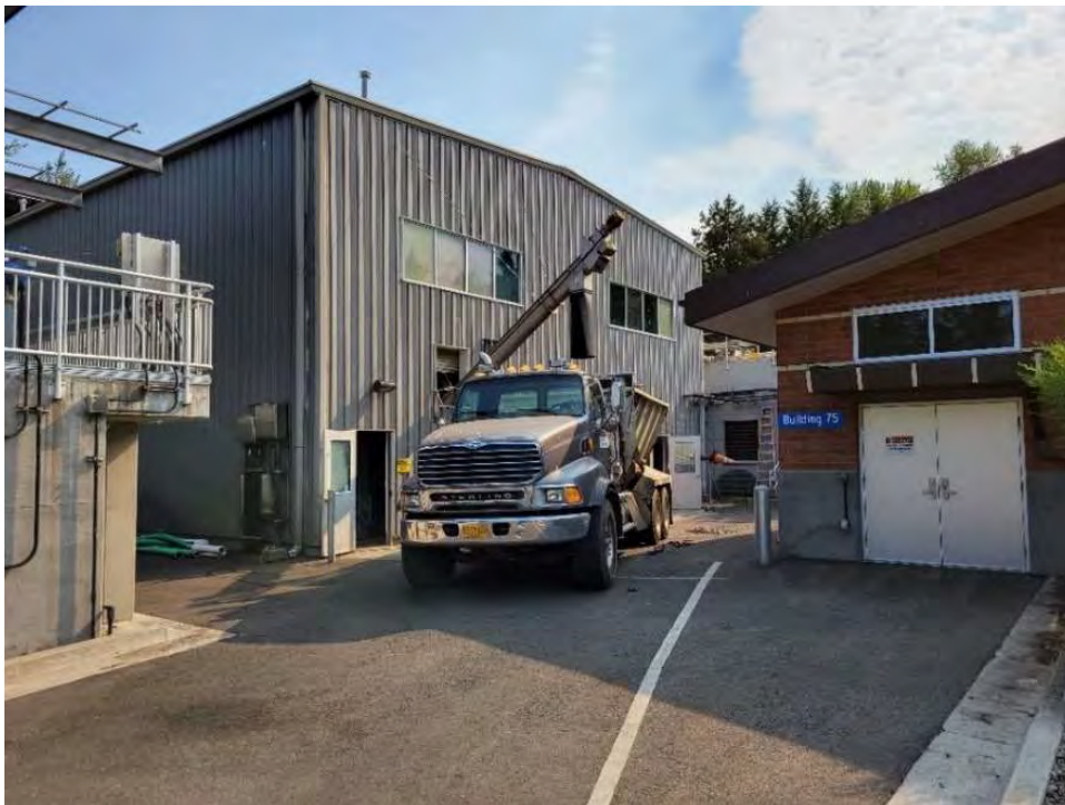
Figure 33. Truck loadout at Solids Handling Building
