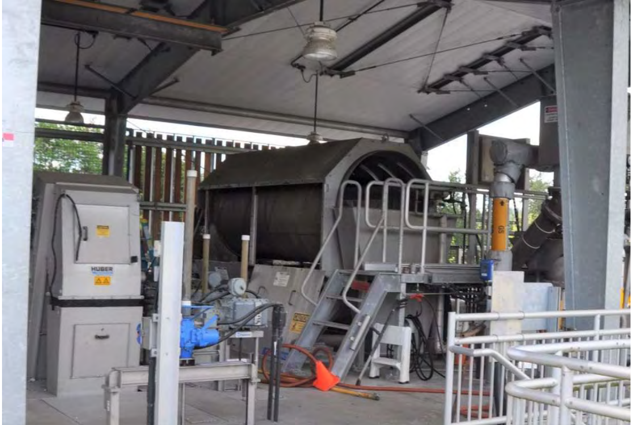
Figure 16. Mixed liquor rotary drum screen
