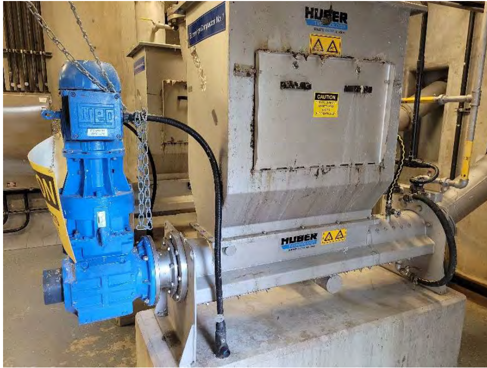
Figure 15. Screenings washer/compactor side view
