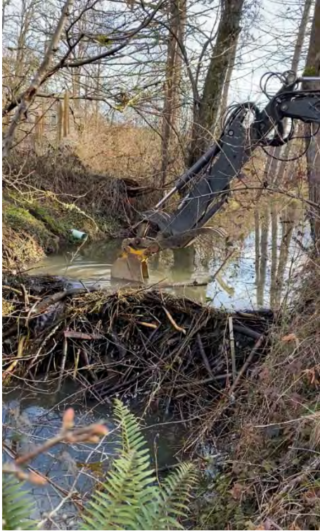
Beaver dam removal
