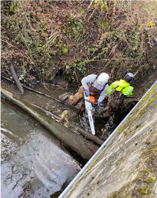
Removing debris from culvert
