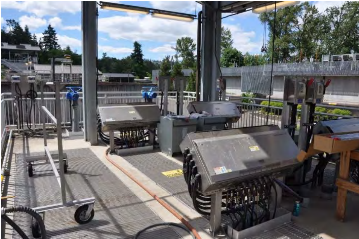
Figure 26. UV channels and equipment photo
