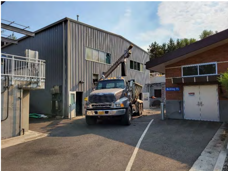
Figure 46. Truck loadout at Solids Handling Building
