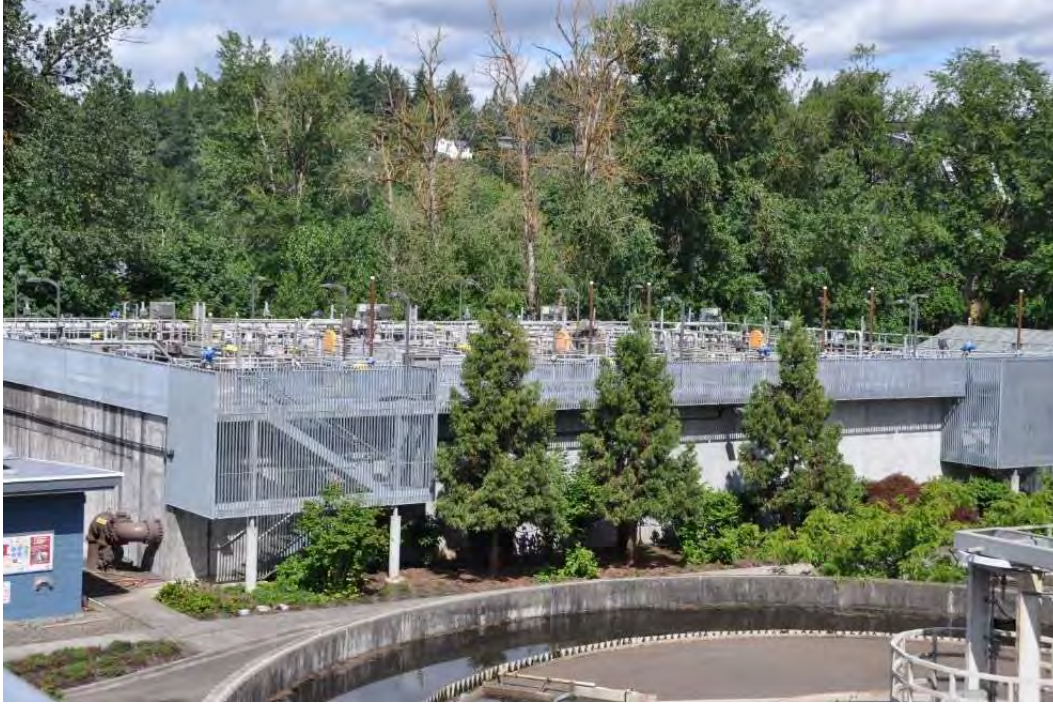
Figure 15. Aeration basin structure
