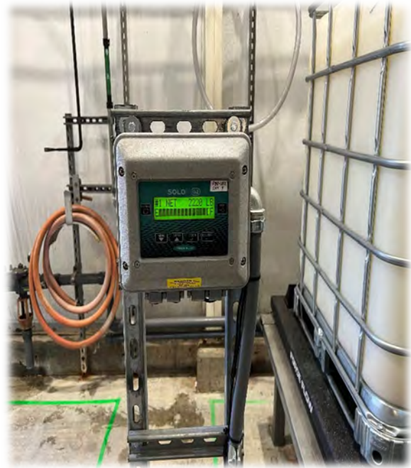
Polymer Scale Installation.
