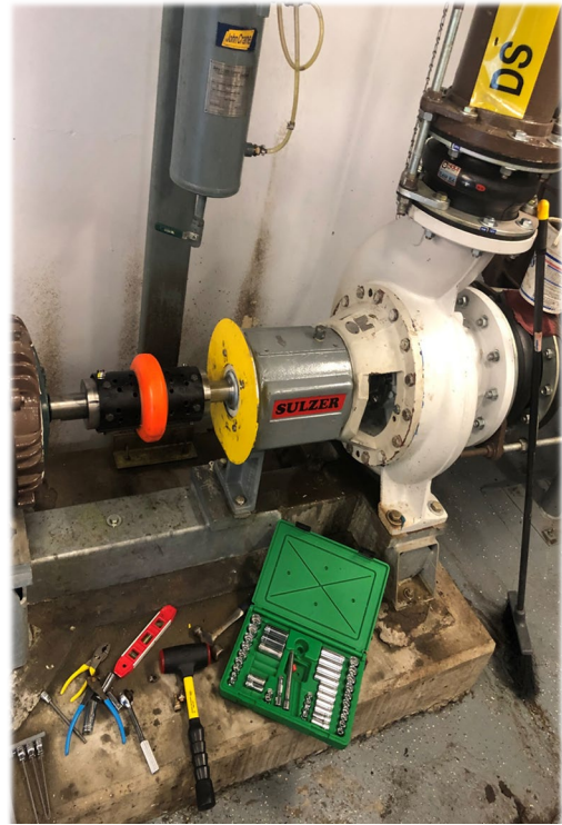
Digester Pump fix with spare
