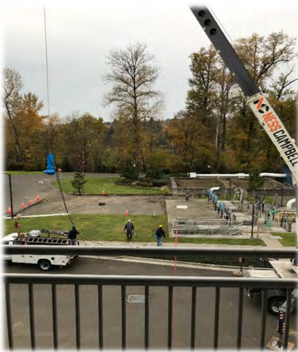
Lifting the second influent pump
