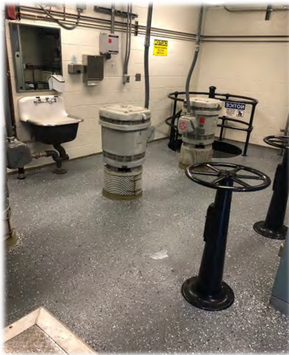
Pump Station #3 floor coating
