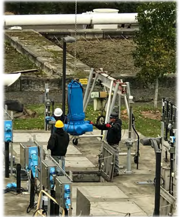
Installing the influent pump
