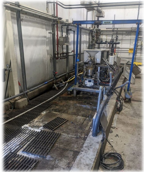
First of the dry systems removed.
