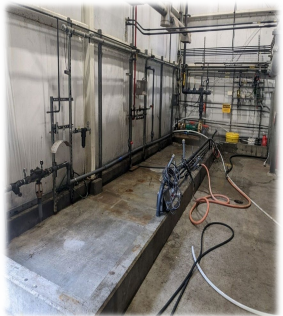
both old systems gone and area cleaned up.
