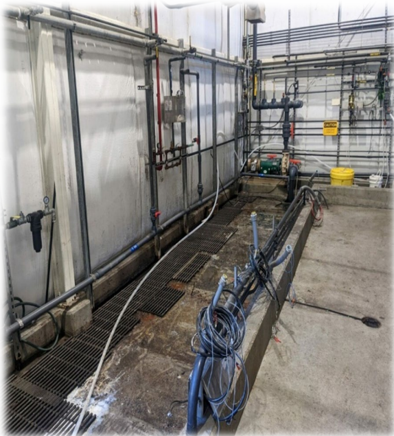
Both dry systems removed.
