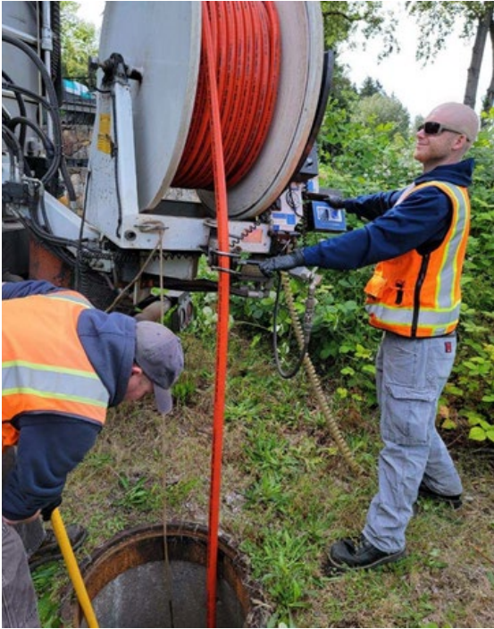
Photo 1: Routine collection system cleaning
