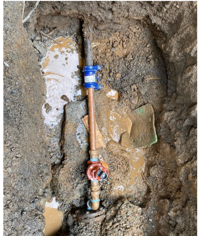
Photo 8: 2-inch galvanized pipe repaired
