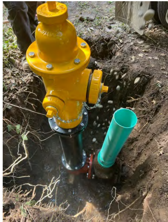
Photo 4: Hydrant replaced on Thornton Dr.
