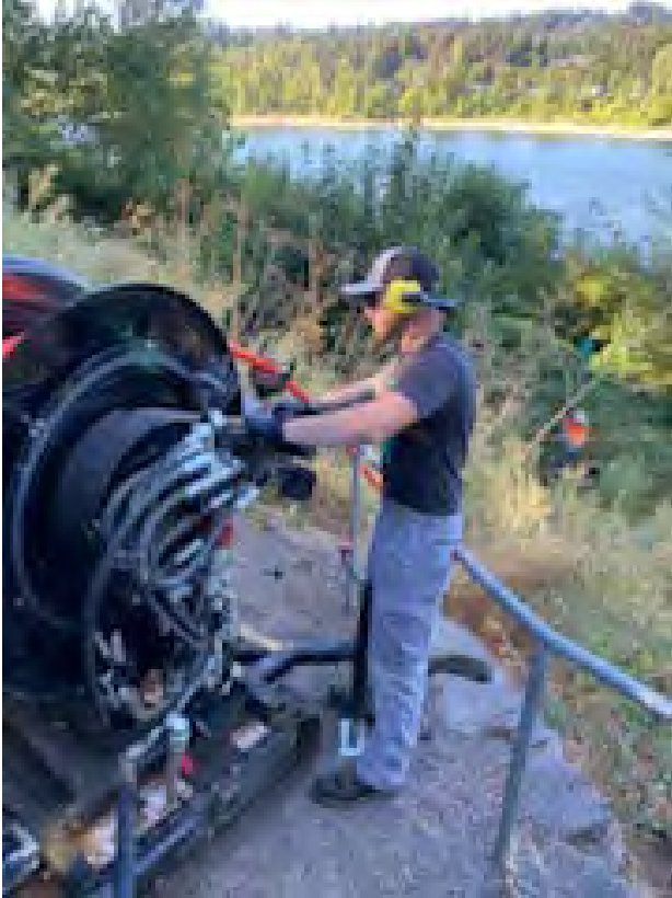
Photo 1: Line segment cleaning using easement machine.
