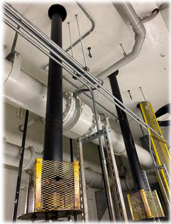
New Drive lines installed at Lift Station #2
