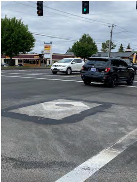
Photo 3: Manhole repair on McLoughlin Blvd. at Roethe Rd.
