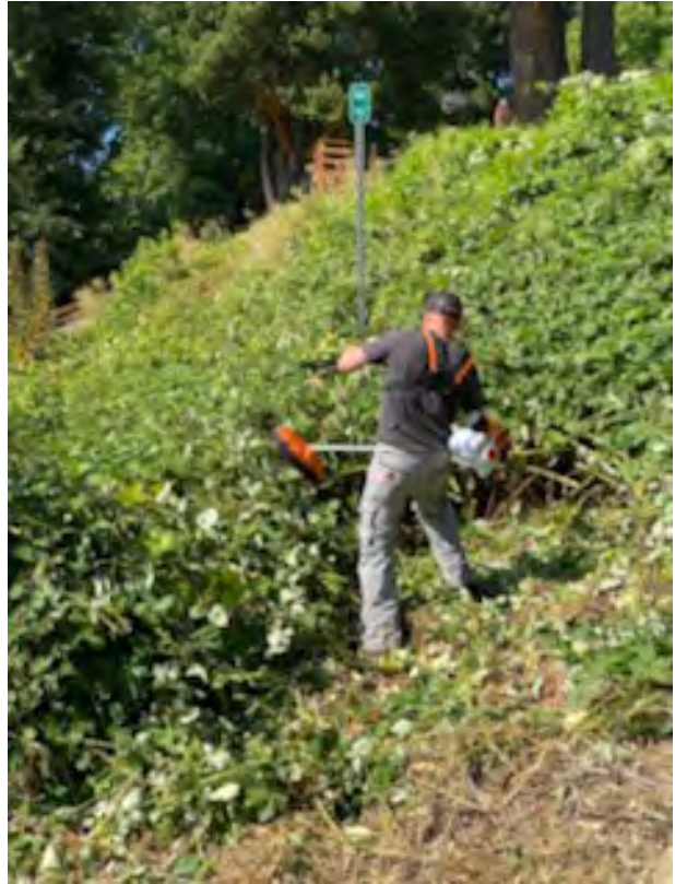
Photo 2: Clearing vegetation to access manhole.
