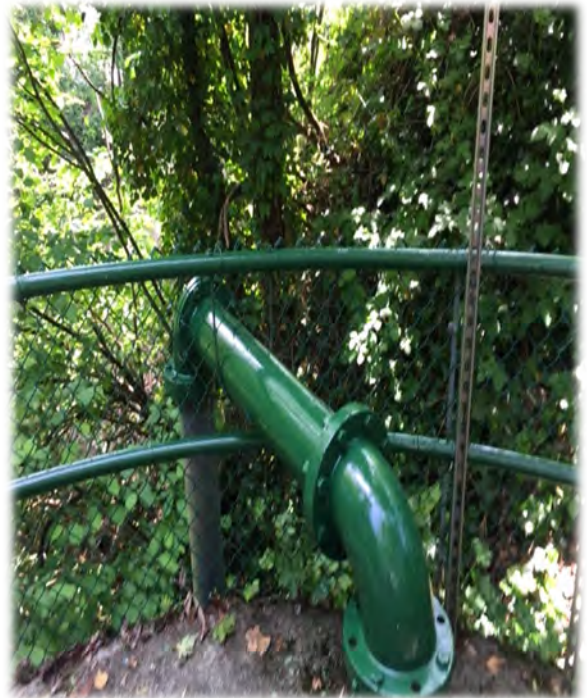
Pump Station #5 after painting
