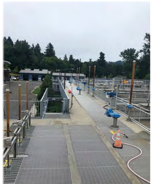
Aeration Basin pressure washed
