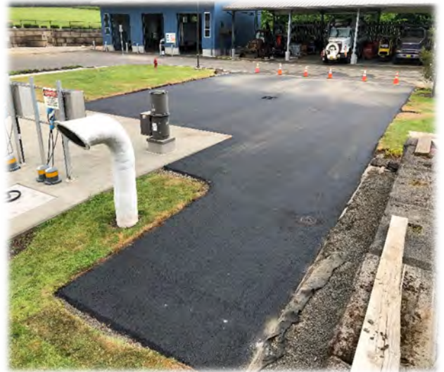
Influent Pump Station Driveway
