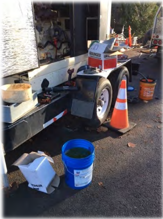
1. Engine generator repair.
