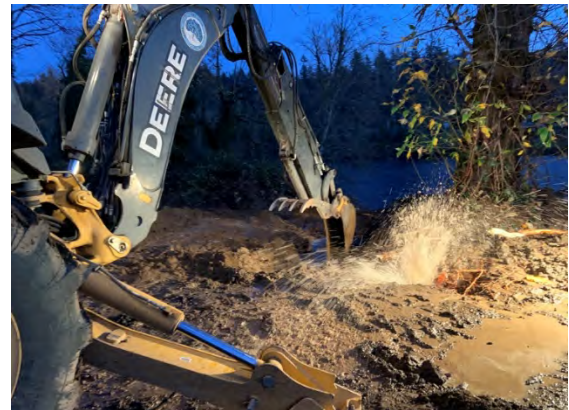
Photo 7: Air relief pipe repair on NCCWC 36-inch main
