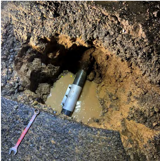
Photo 6: River Road at Oak Shore Lane
