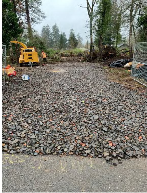
A properly constructed construction entrance
