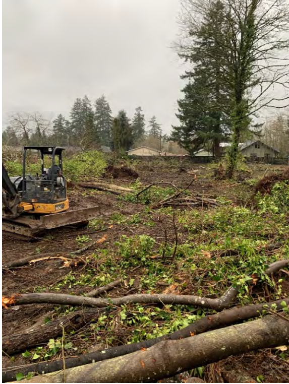
Common Site Clearing of a sub-division
