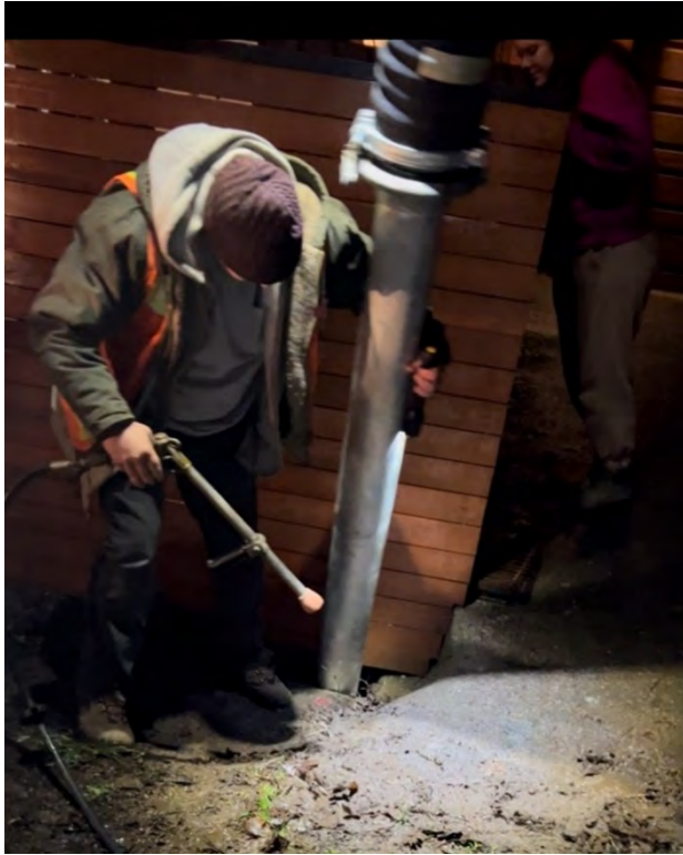
Photo 1: Urgent catch basin clearing on Christmas Eve
