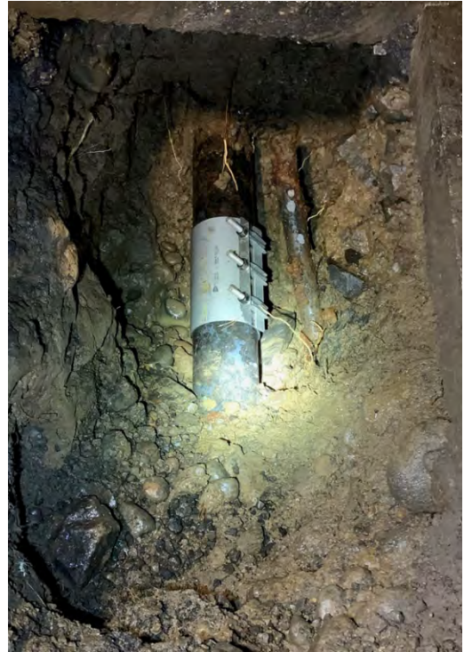
Photos 4 & 5: Crieghton Ave. leak repair
