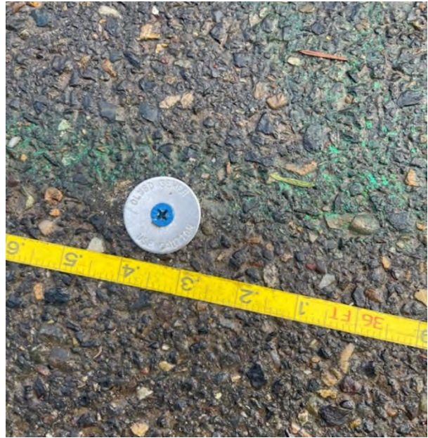
Photo 2: Locating pin installed in asphalt
