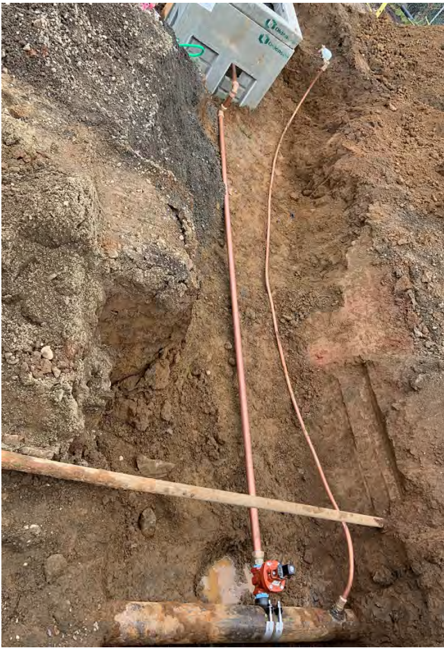
Photo 5: Water service installations on Cedar Ave.
