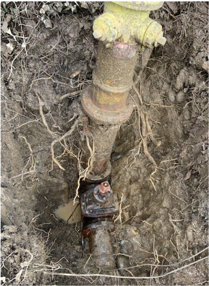
Photo 6: Fire hydrant prior to rebuild on Laurie Ave.
