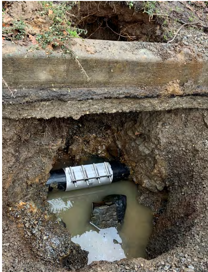
Photo 9: Main leak repair on McLoughlin Blvd.
