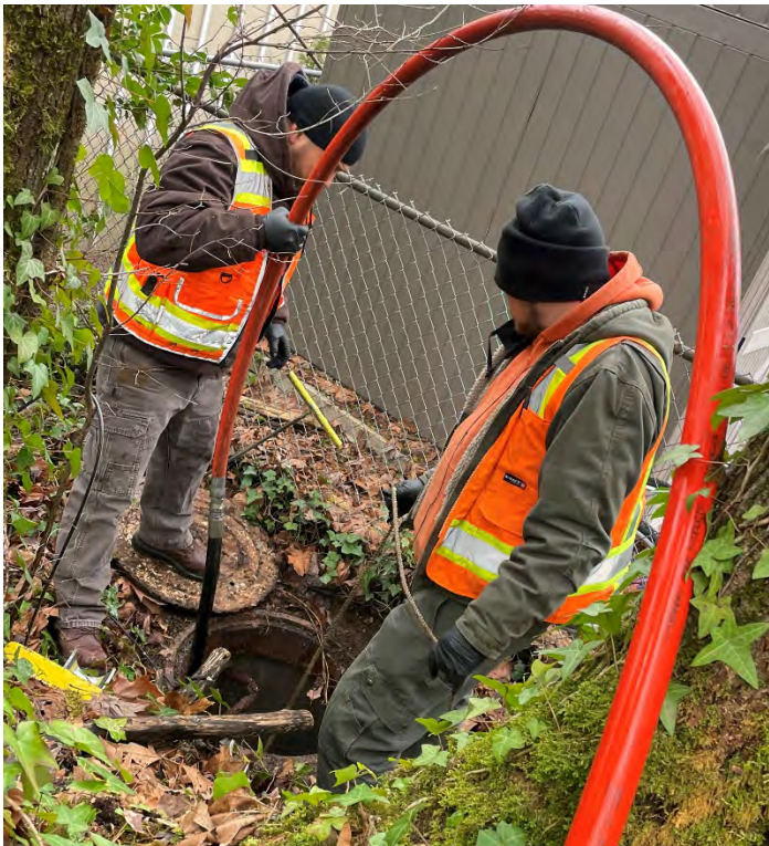
Photo 3: Cleaning underway through manhole on private property
