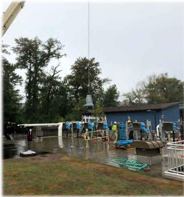
Installation of new IPS pumps
