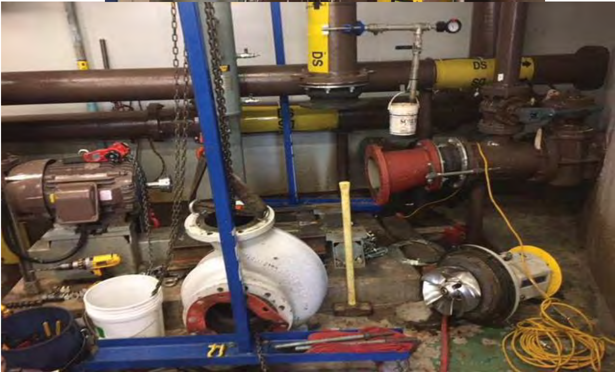
Photos 1&2 Creative lifting devices in tight locations
