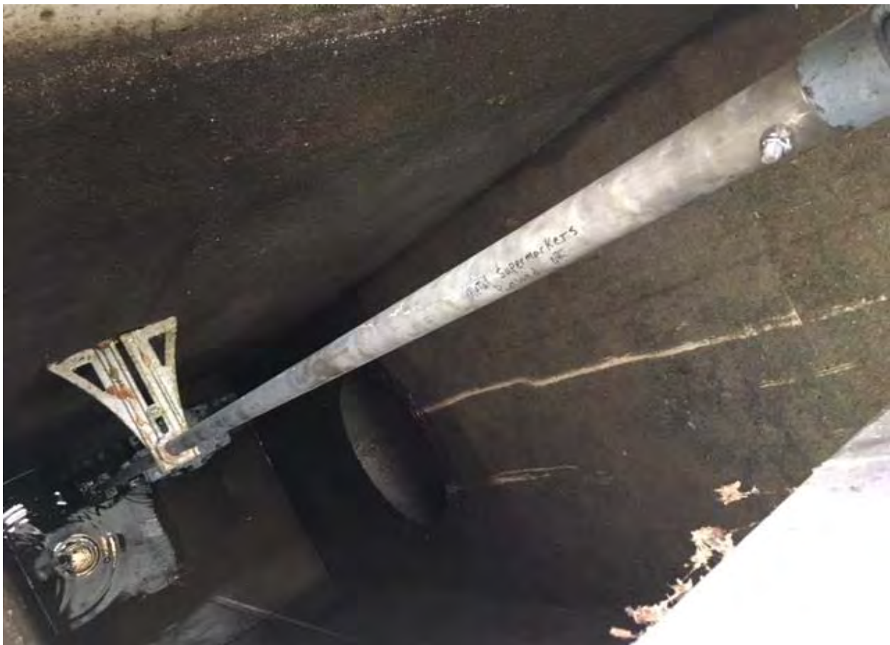
Photo 9&10 The bracket where the shaft broke and the new shaft installed.
