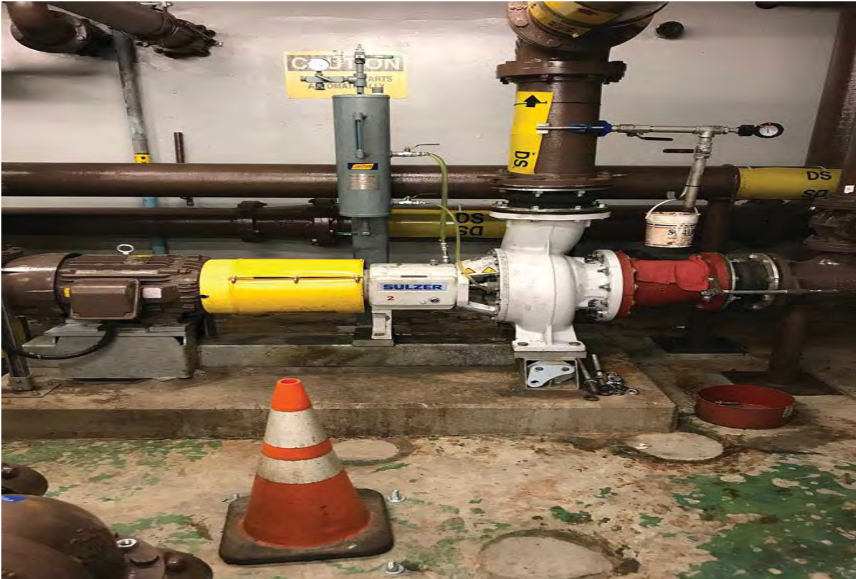
Photo 3&4 Installation of volute and final product: Digester pump #2
