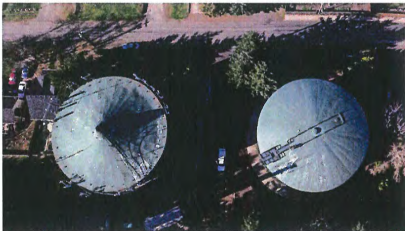
This picture shows both tanks located at 4412 SE View Acres Rd. the tank on the right is the proposed location.
