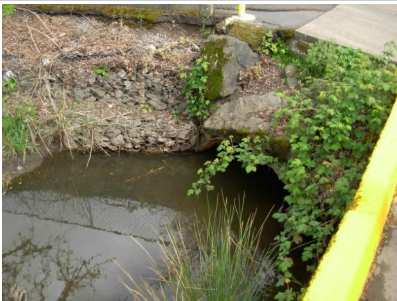
Site location: 015 Photo number: 046 Description: Downstream end of culvert under Boardman Ave.
