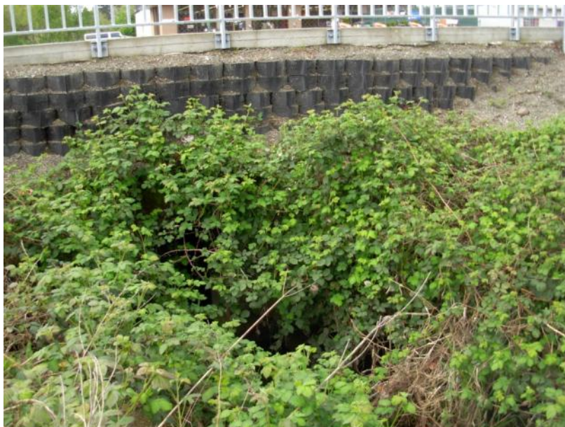
Site location: 015 Photo number: 047 Description: ODOT keyhole culvert under 99E.
