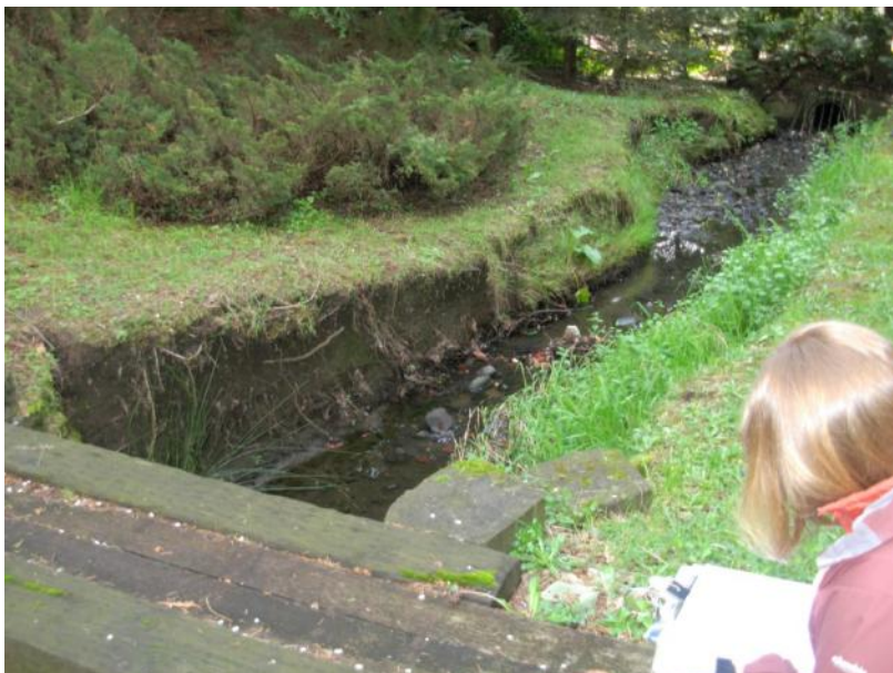
Site location: 012 Photo number: 034 Description: Private Property (3320 West View Ave).
