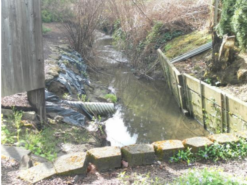
Site location: 001 Photo number: SAM_1189 Description: Public ROW - Upstream of culvert under SE Laurie Ave (15300 SE Laurie Ave.)
