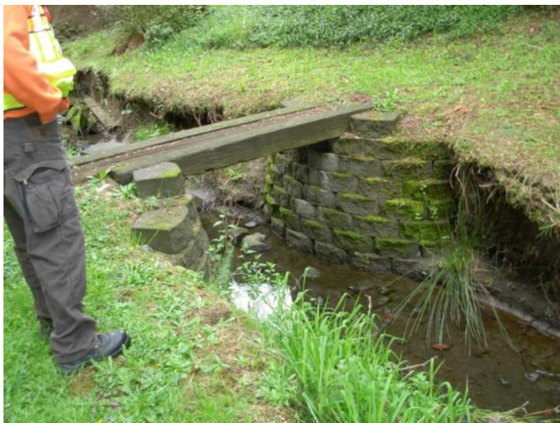
Site location: 013 Photo number: 037 Description: Private Property (3320 West View Ave).
