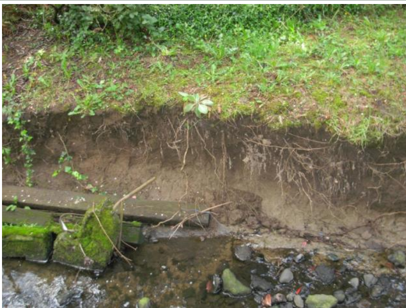
Site location: 012 Photo number: 033 Description: Private Property (3320 West View Ave).
