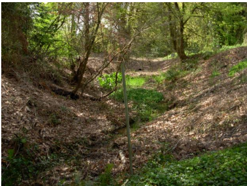
Site location: 011 Photo number: 028 Description: Widened channel downstream of SE Linden Ave. Discharge to culvert under SE Linden Avenue.
