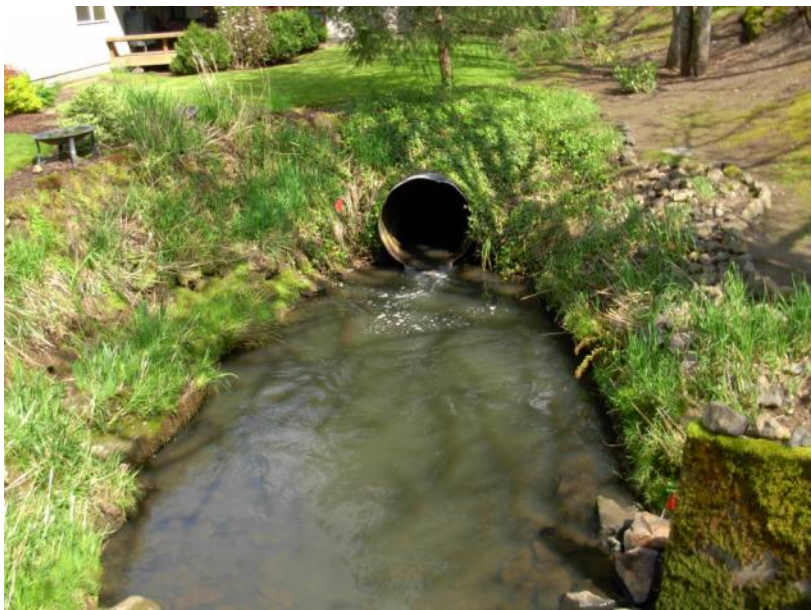
Site location: 021 Photo number: 062 Description: Public ROW – Boardman Creek discharge from culvert under River Rd.
