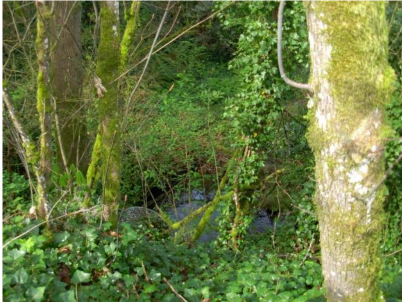
Site location: 010 Photo number: 019 Description: Downstream of culvert under River Road.
