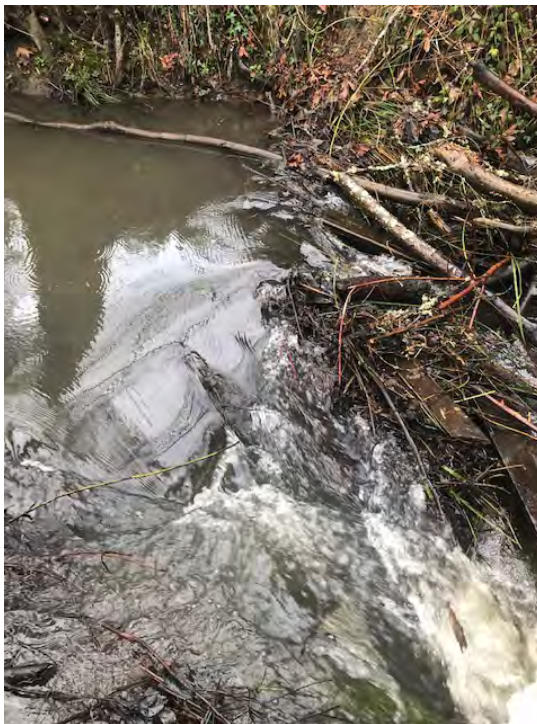
Beaver Dam Removal (1/8/20)
