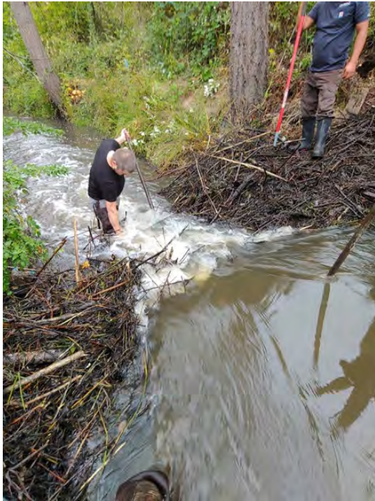
Beaver Dam Removal (9/23/20)
