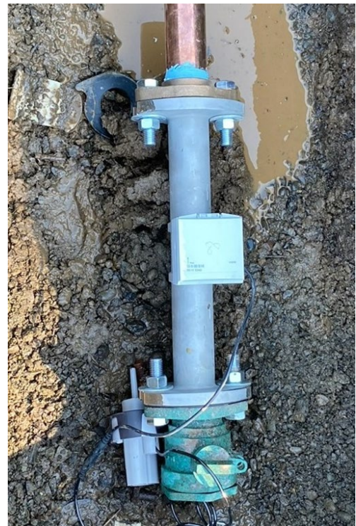
Photo 4: 2-inch meter exchanged on Boardman Ave.
