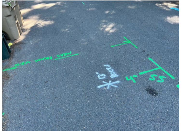
Photo 2: Underground utility locate work
