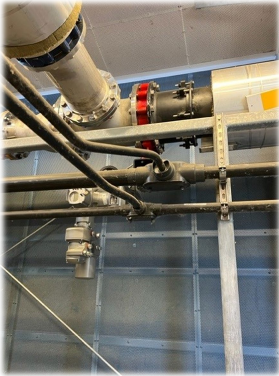
New Valve Installation on blowers
