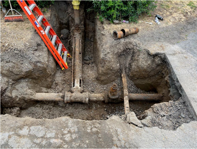
Photos 5 & 6: Fire hydrant, tee, and valve replacement on Arista Drive
