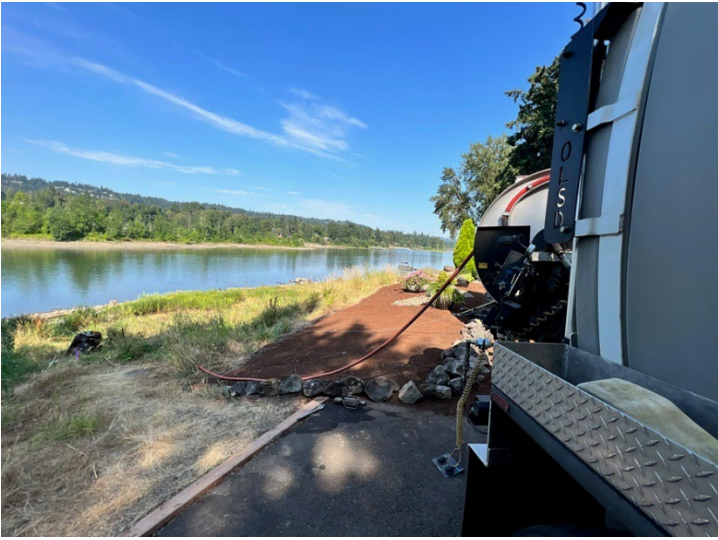
Photo 1: Hydrocleaning on Willamette Drive
