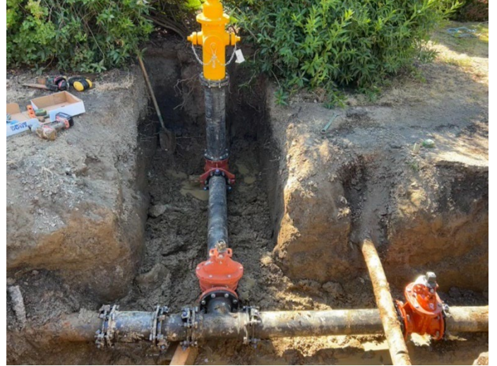
Photos 5 & 6: Fire hydrant, tee, and valve replacement on Arista Drive
