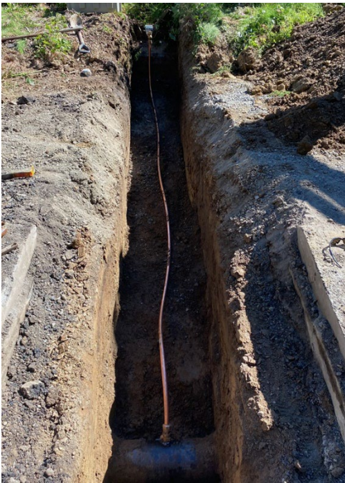
Photo 7: New service installation on Aldercrest Road
