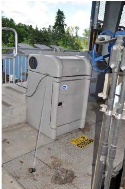
Figure 8. Influent composite sampler
