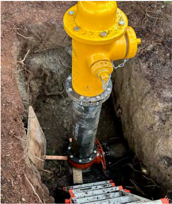
New hydrant install Roethe Road
