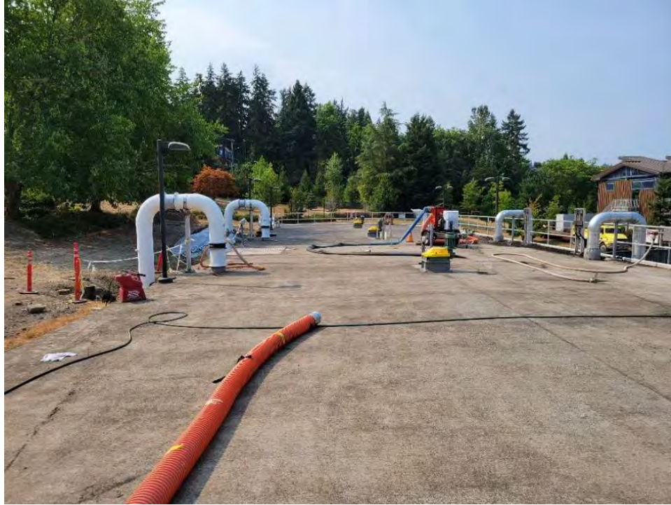
Figure 36. Top of Aerobic Digesters 1 and 2
