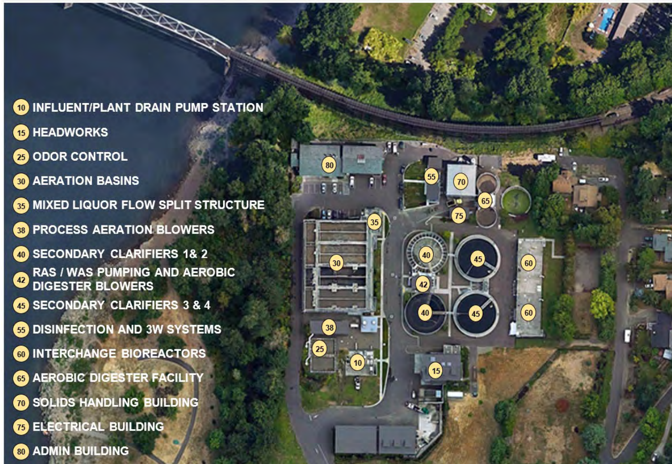
Figure 2-5. Aerial view of WWTP with major facilities labeled
