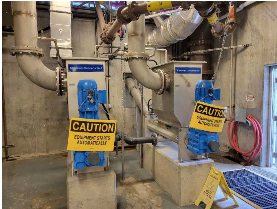
Figure 14. Screenings washer/compactors
