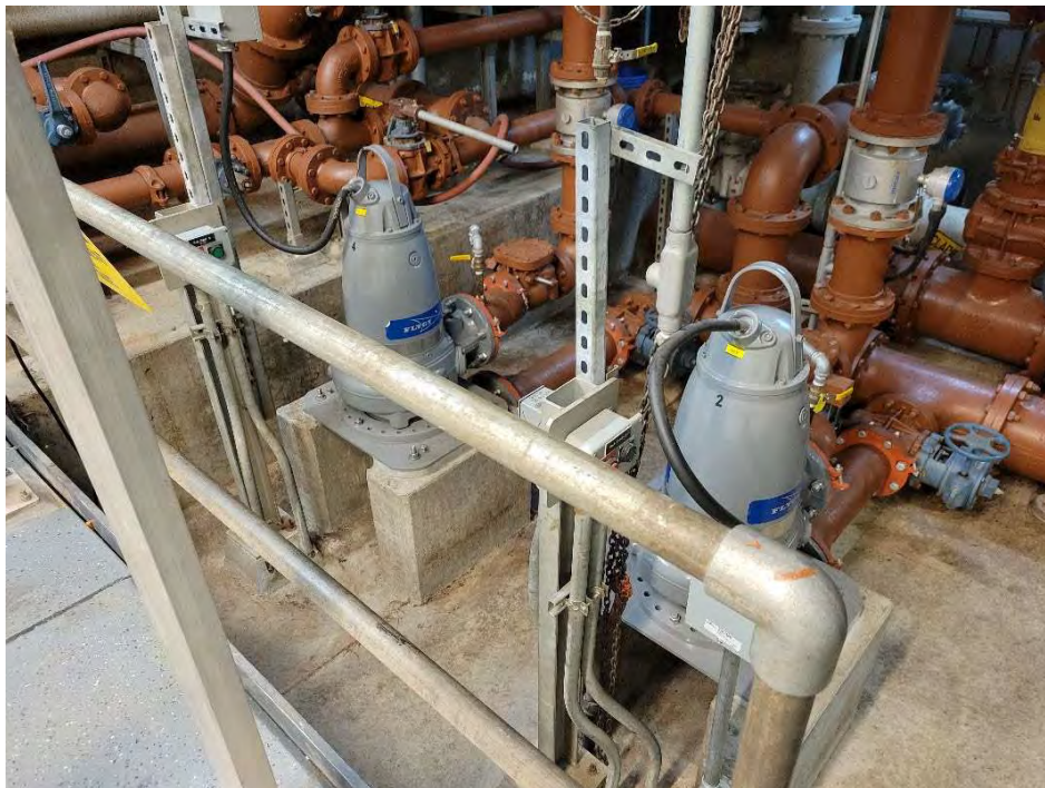
Figure 31. West RAS pumps in RAS/WAS pump station
