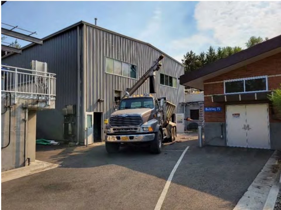
Figure 33. Truck loadout at Solids Handling Building
