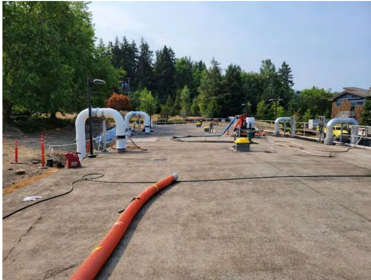
Figure 28. Top of Aerobic Digesters 1 and 2
