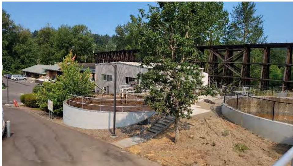
Figure 29. Circular aerobic digester
