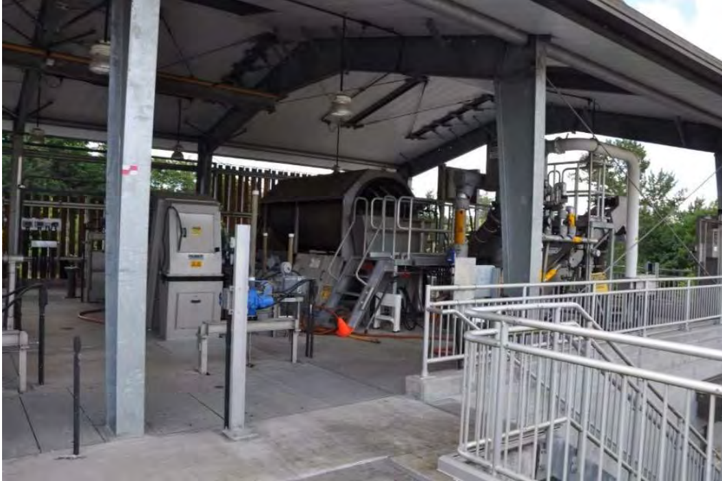
Figure 13. Mixed liquor rotary drum screen
