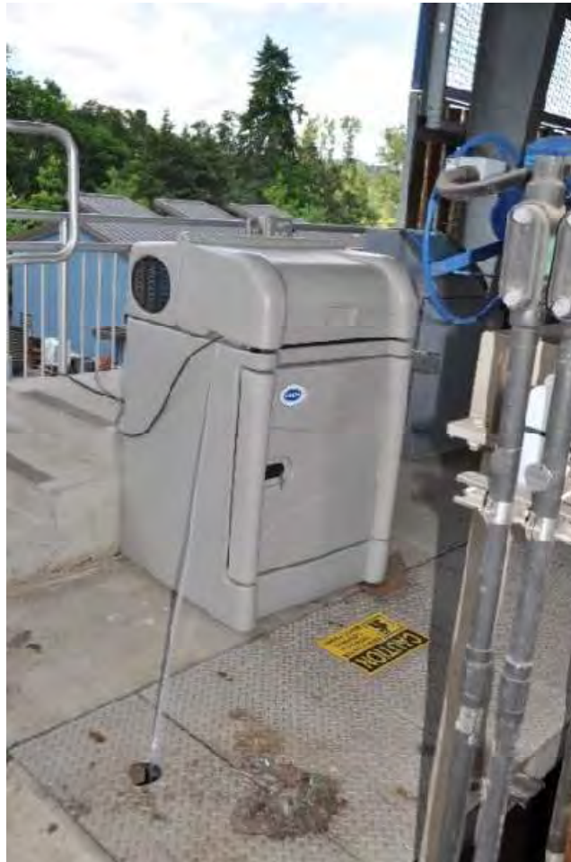
Figure 9. Influent composite sampler
