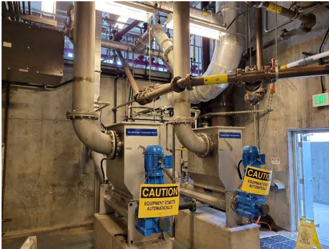
Figure 12. Screenings washer/compactors
