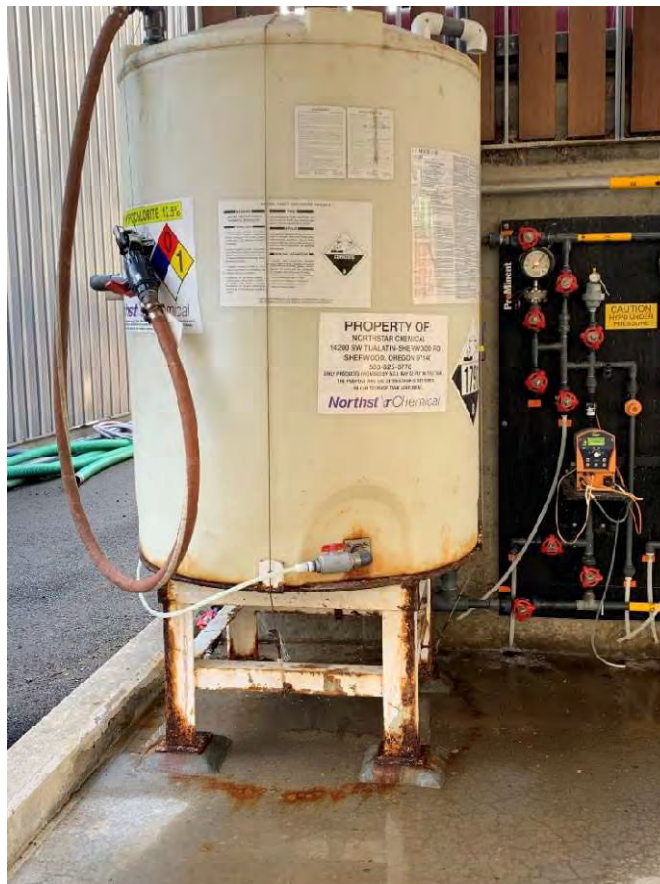
Figure 49. Sodium hypochlorite storage tank
