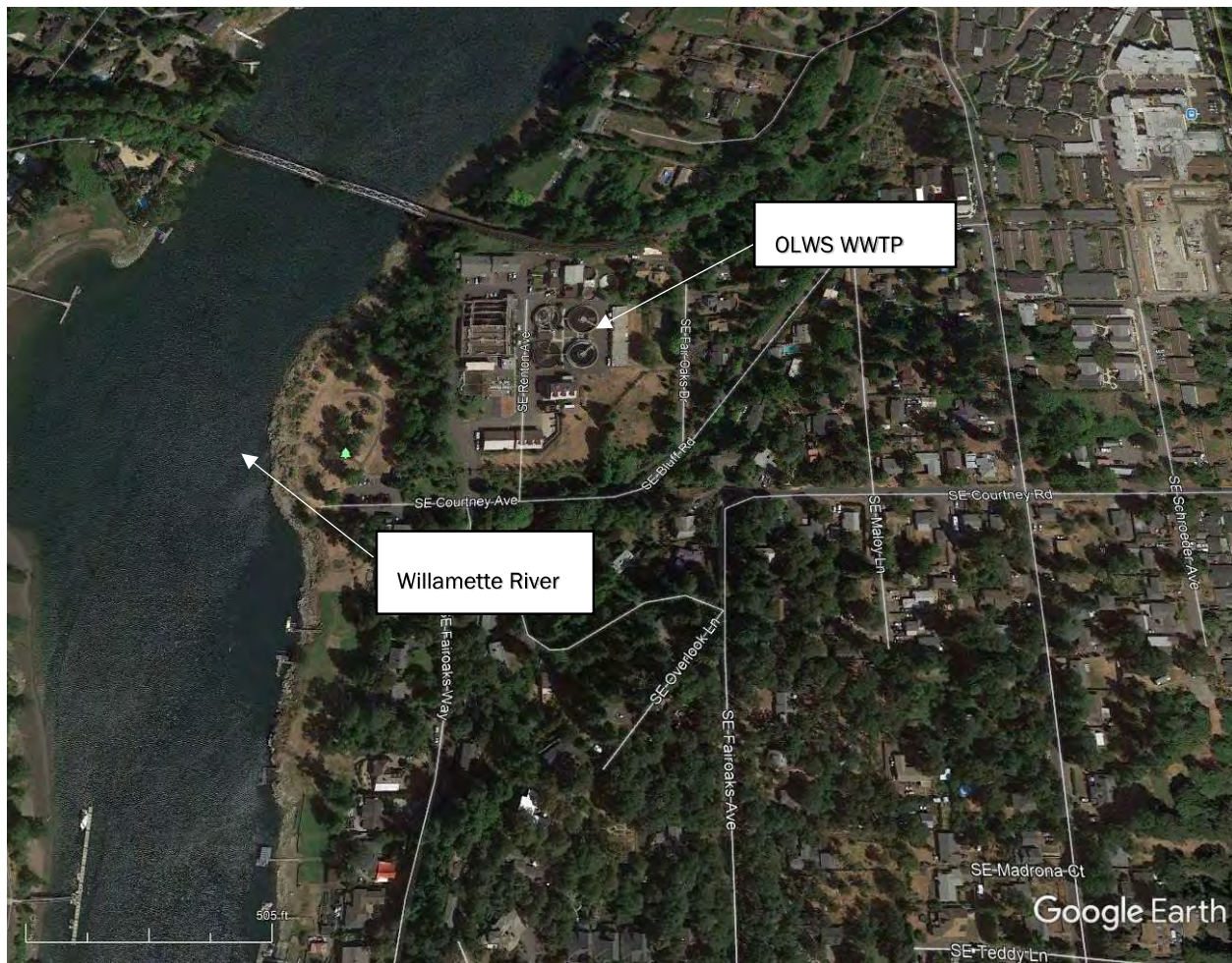
Figure 1. OLWS WWTP aerial photo
