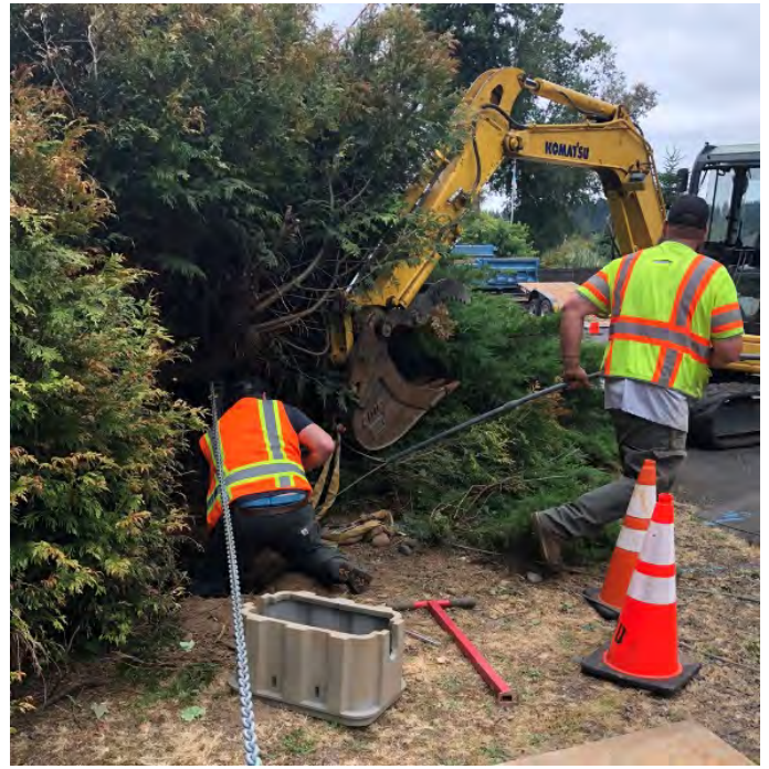
6. Service line repair at wastewater Pump Station 2
