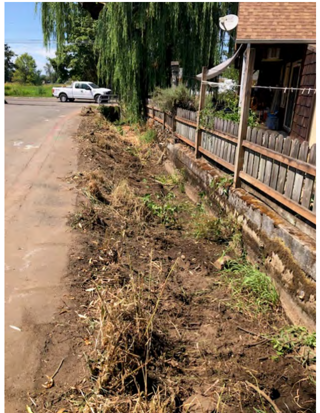
8. After prep work (looking north)
