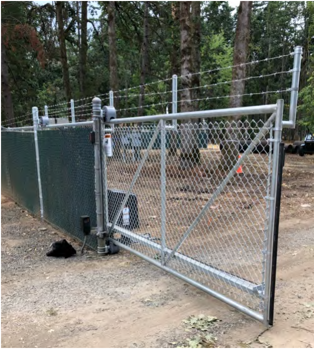
5. New gate at Valley View
