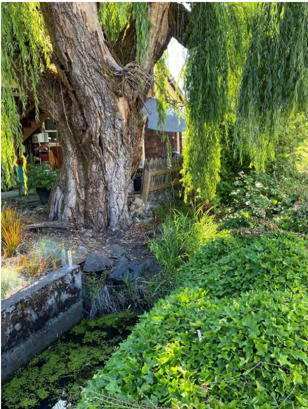
7. Boardman open channel prior to prep work (looking south)
