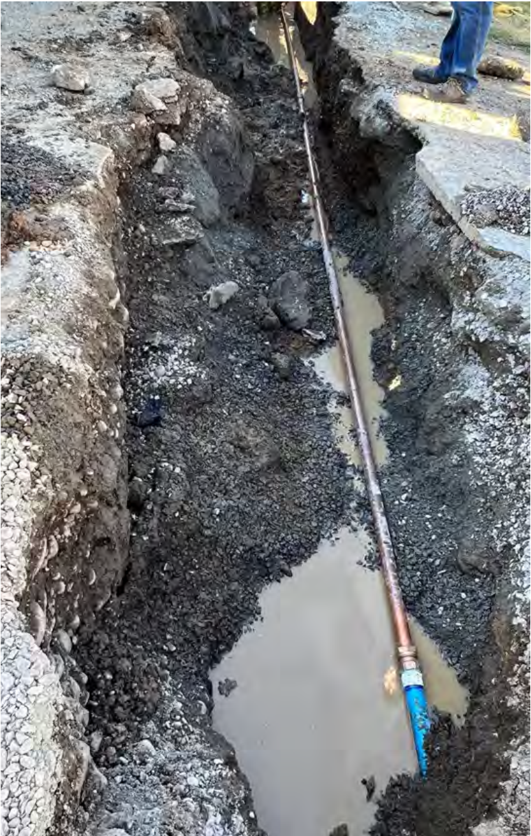
Photo 6: New copper tubing installed
