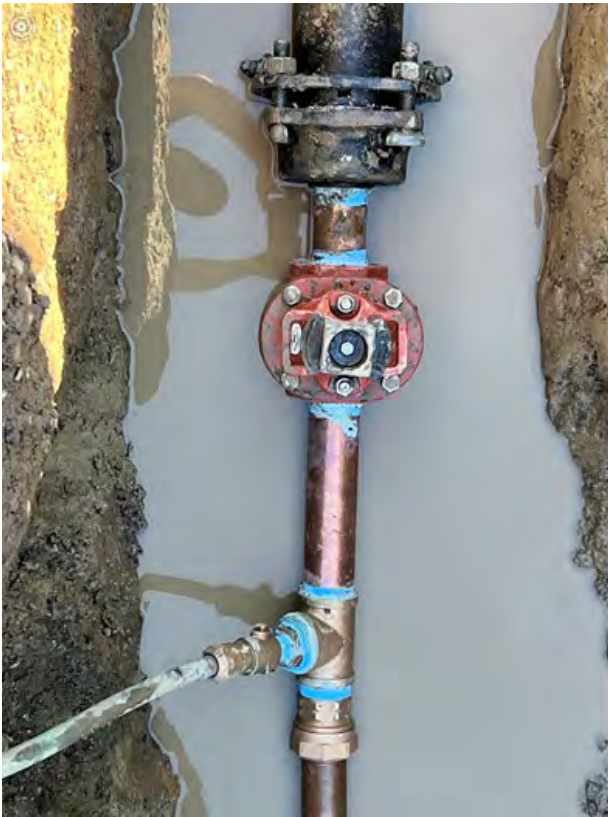
Photo 7: Tie-in point of new 2-inch copper
