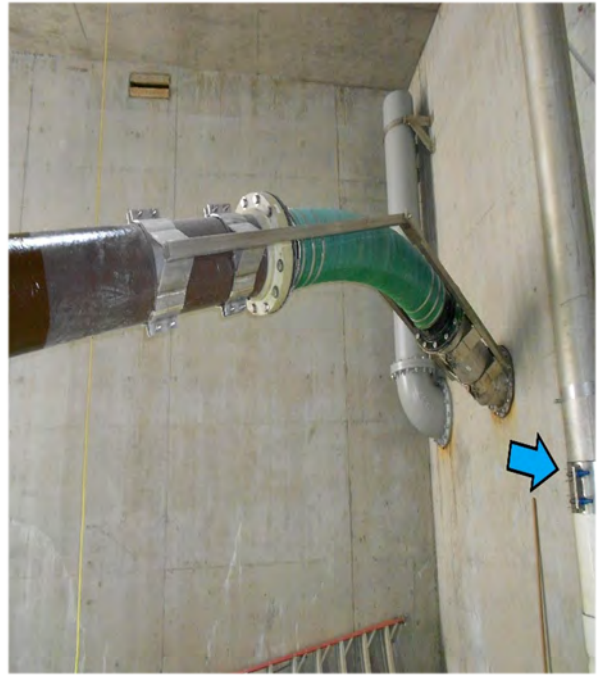
Different Angle of Suspected Bad Clamp
