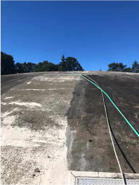
(1) Picture of South reservoir dome, after pressure washing.
