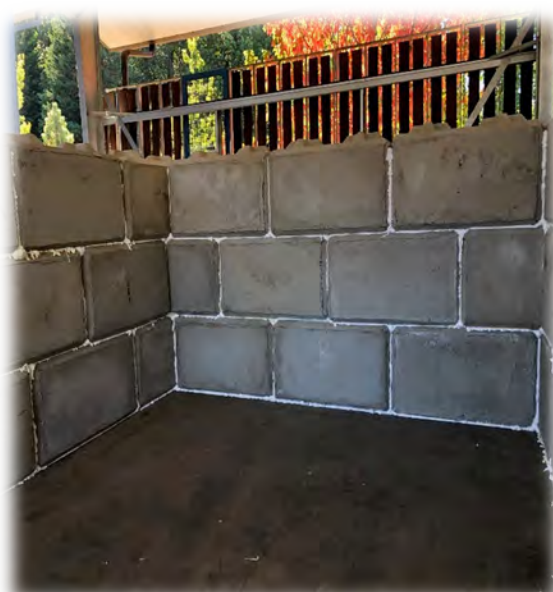
4) Biosolids storage complete
