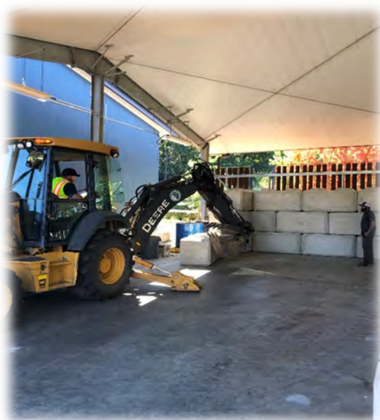
3) Construction of biosolids storage
