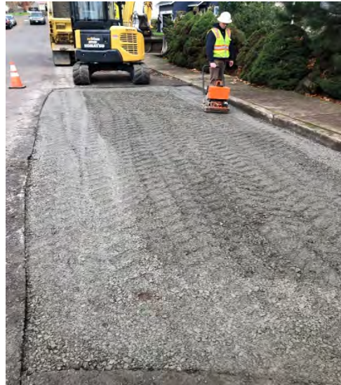
Photo 4: Temporary roadway patch at Hull & Rose
