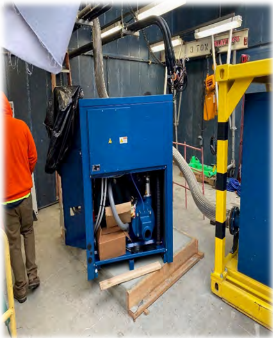
Aerzen Process Blower #2 Being Seated.
