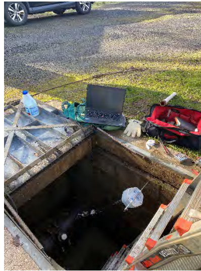
16" Water Meter Test
