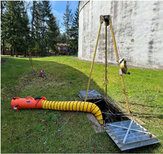
24" Water Meter Test
