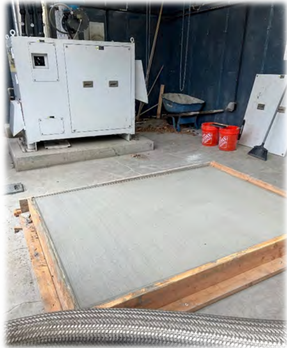
New Pad Poured for Process Blower #2.
