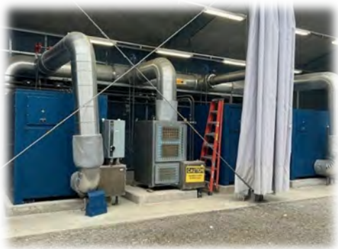
New blower install (third from left).
