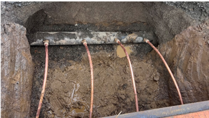
Above - New services on Ina Ave.
