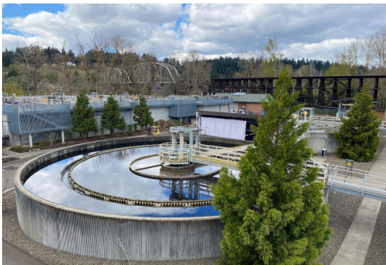
Wastewater Treatment Plant 13750 SE Renton Avenue Oak Grove, OR 97222
